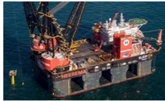
Installing the 395t P-11 Unity platform
