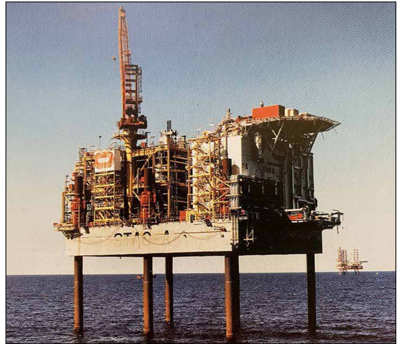
The Central Production Facility EPC contract for Apache's Stag field was won by Bouygues Offshore. It was based on a design that was self-installable and reusable. It was transported to site by the submersible vessel Mighty Servant 3.
