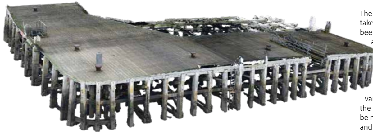
A broadscale reconstruction of Helensburgh pier, combined from aerial and sub-tidal surveys, made to map the underwater structure of the pier and the areas of damages caused by collisions and fire.
