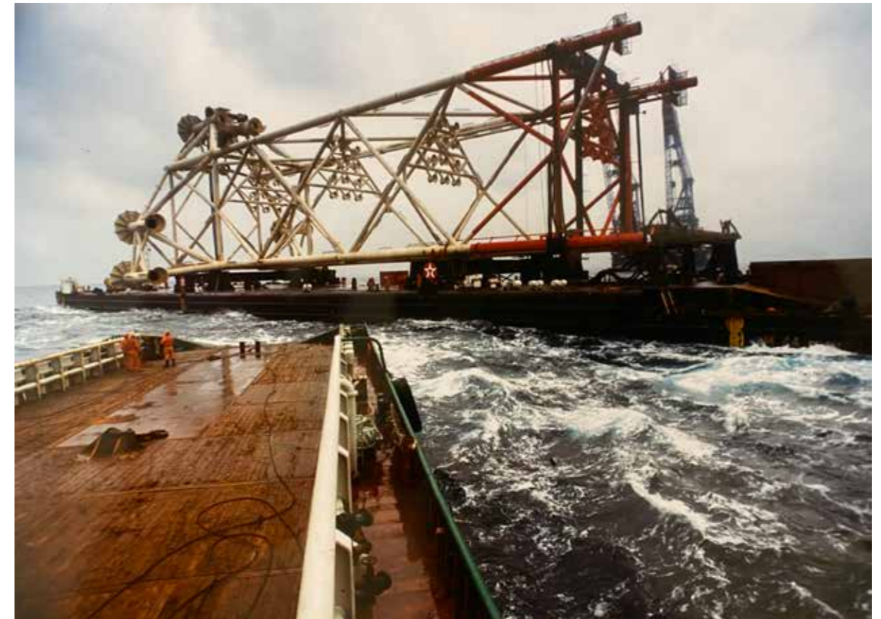
The 2720t Erskine jacket on the Saipem M-44 barge prior to its installation in the field by the Saipem S7000 heavy lift vessel
