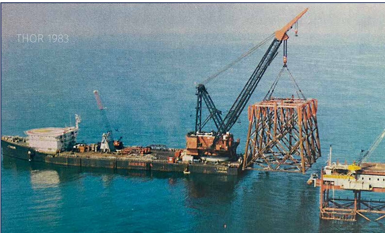
Heerema's Thor barge installing part of the gas compression platform on the Inde gas field -at the time, the largest gas compression project in the world.
