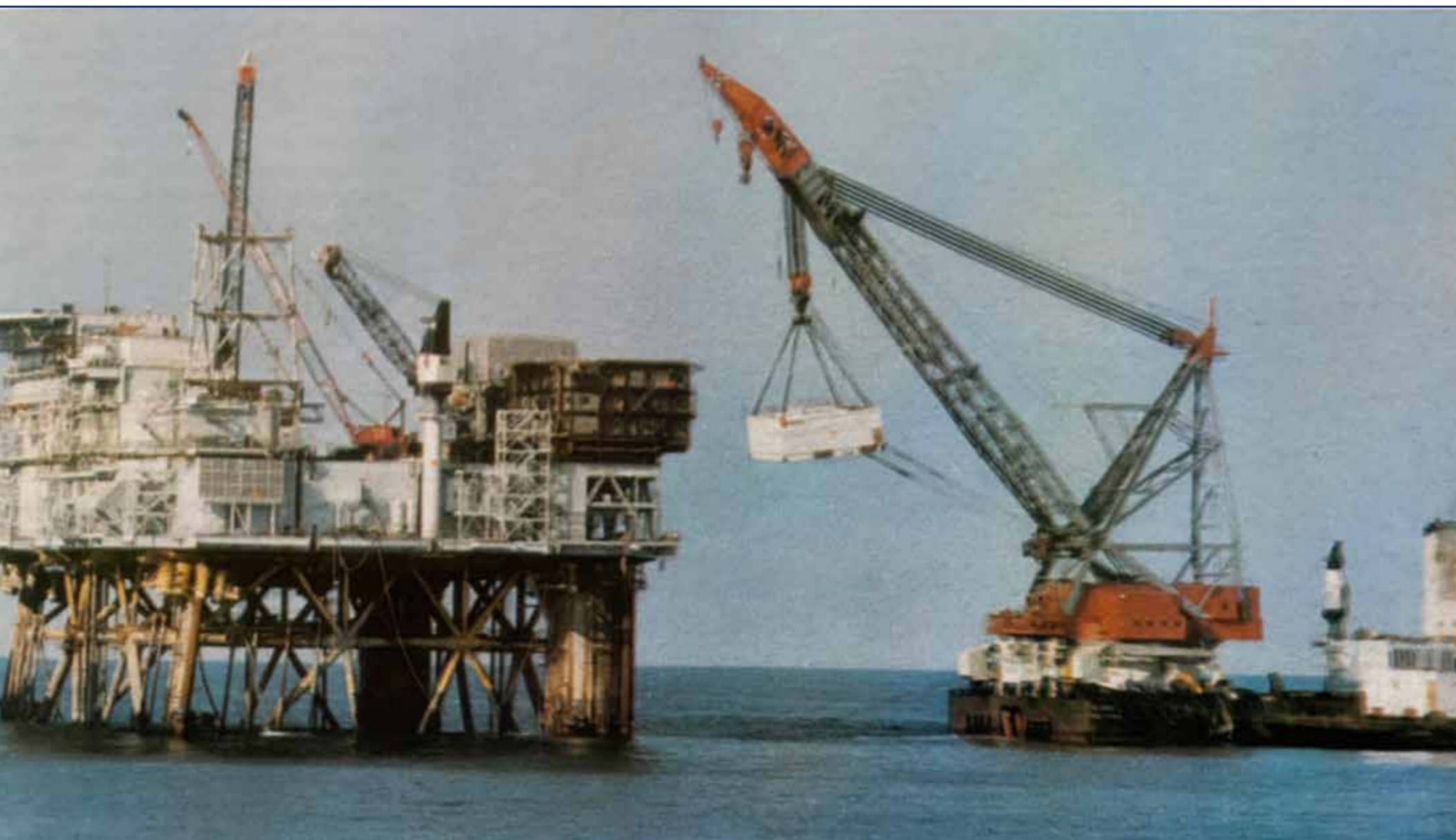
Offshore cranes are able to lift enormous integrated decks onto jackets. This was not always so.
