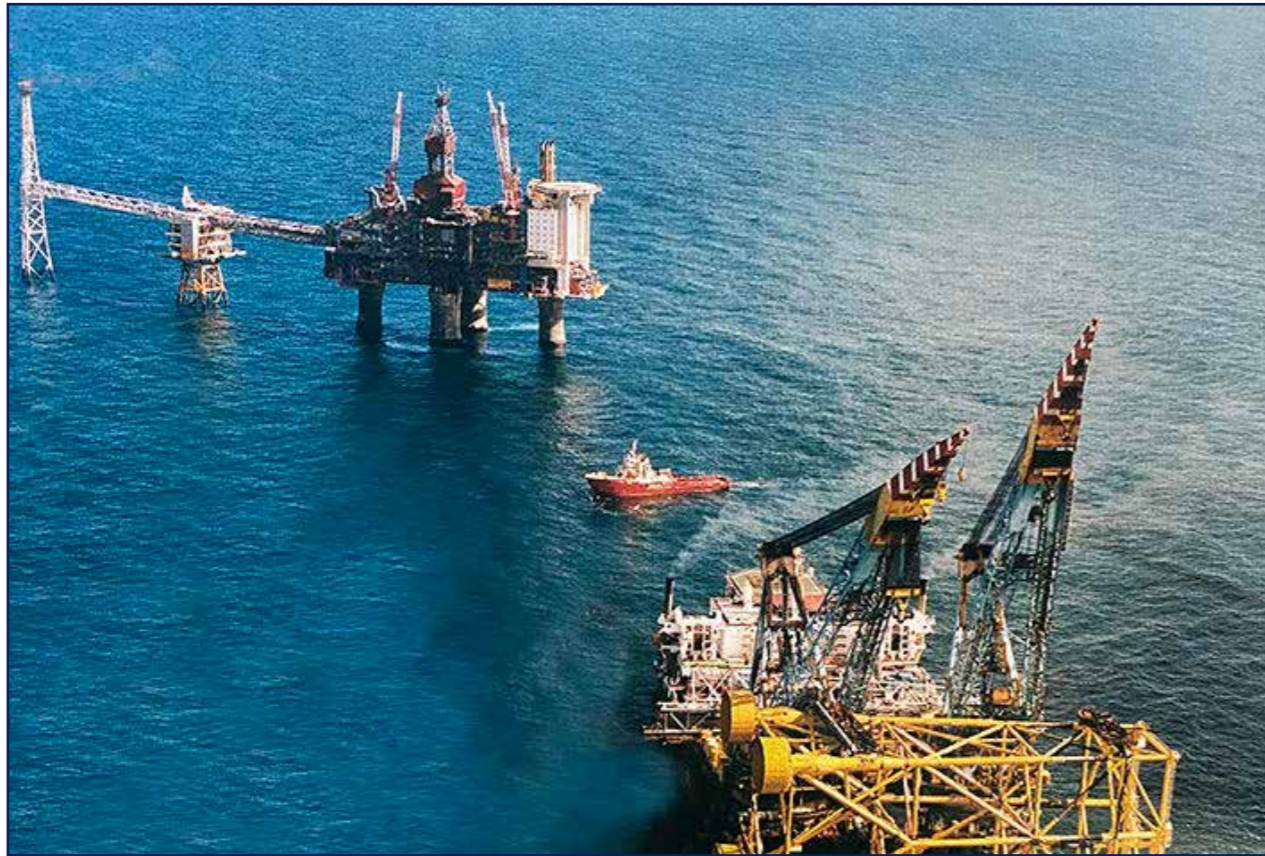
The installation of the jacket on Sleipner T by the S7000. On the left is the slightness a concrete platform bridge-linked to the riser platform and flare structure. At the base of the jacket are 14 m diameter suction buckets
