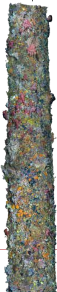
A 3D model of coral coverage on an oil platform leg at 40+ metres depth in the Gulf of Thailand. The model was generated from ROV video of opportunity.
