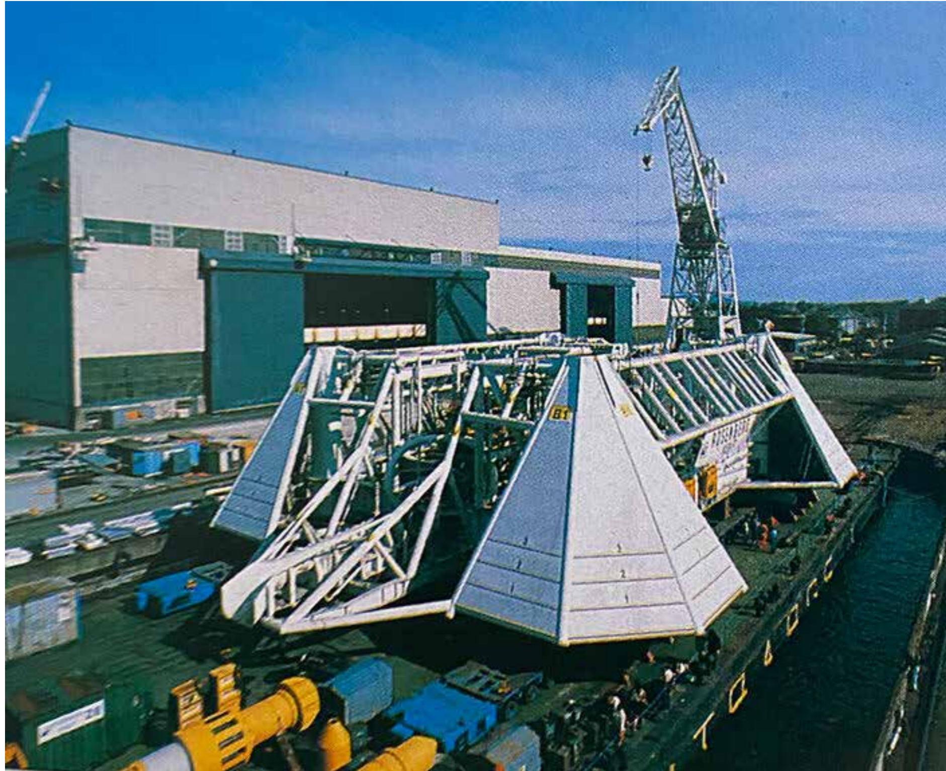
A diverless subsea station installed in 305 m of water to collect and produce from five gas wells on Troll East. The gas was transported to Oseberg for pressure maintenance and increased oil recovery
