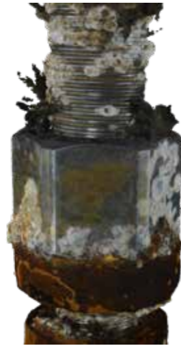
insert (below left) showing close up detail invested recently in new compact through-water GPS equipment that supports accurate georeferencing of the models.
