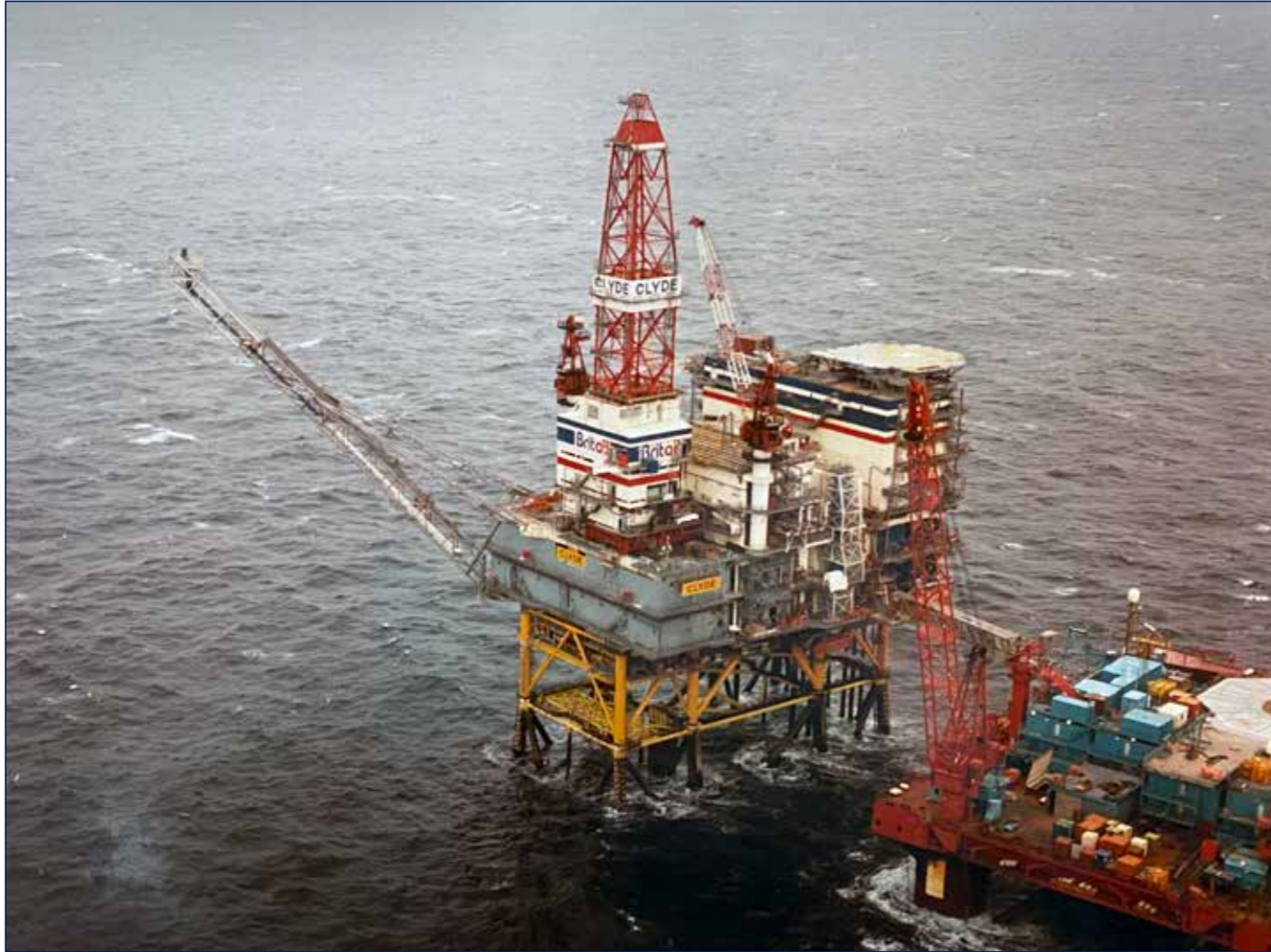
Britoil's Clyde with the Safe Gothia alongside carrying out hook up and commissioning
