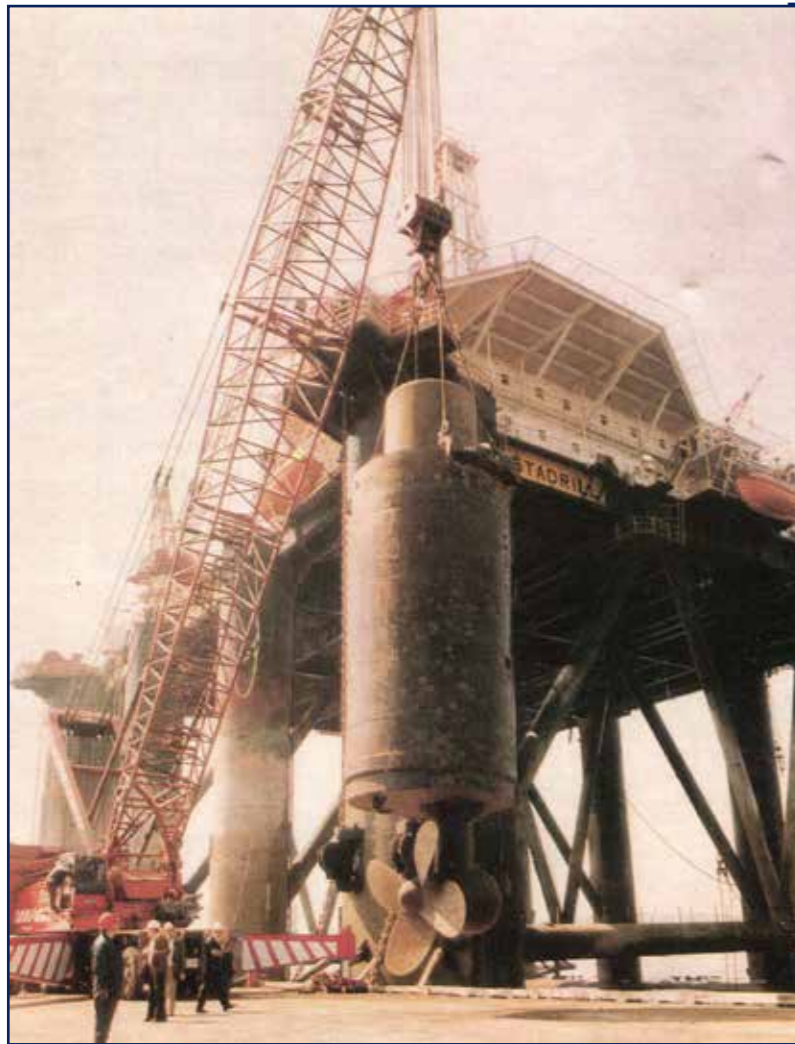
At the BOC base in Peterhead during annual inspection. The pic shows the bow thruster being lifted out.
