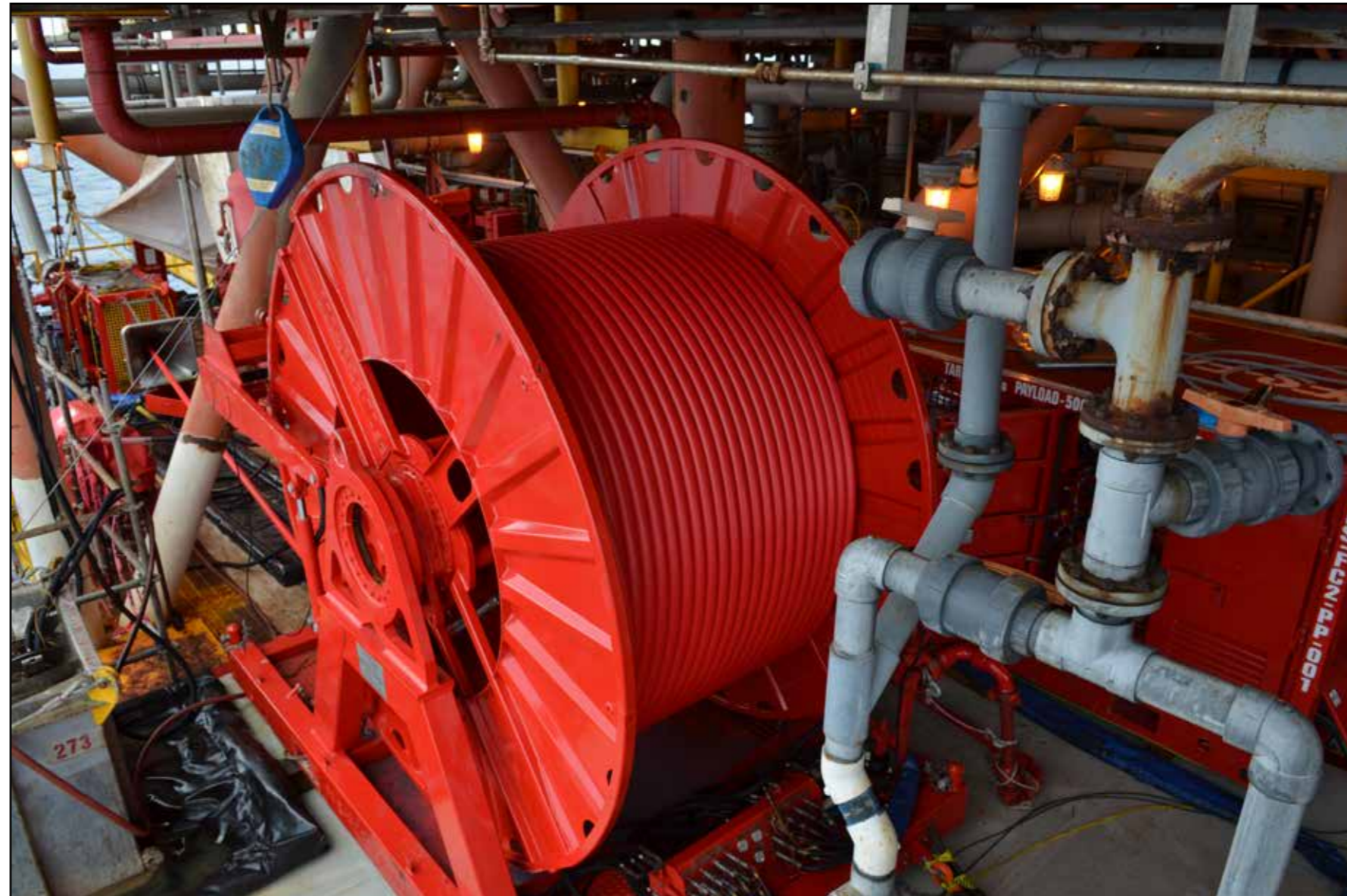
Flexi-Coil deployed under-deck in a very congested area
