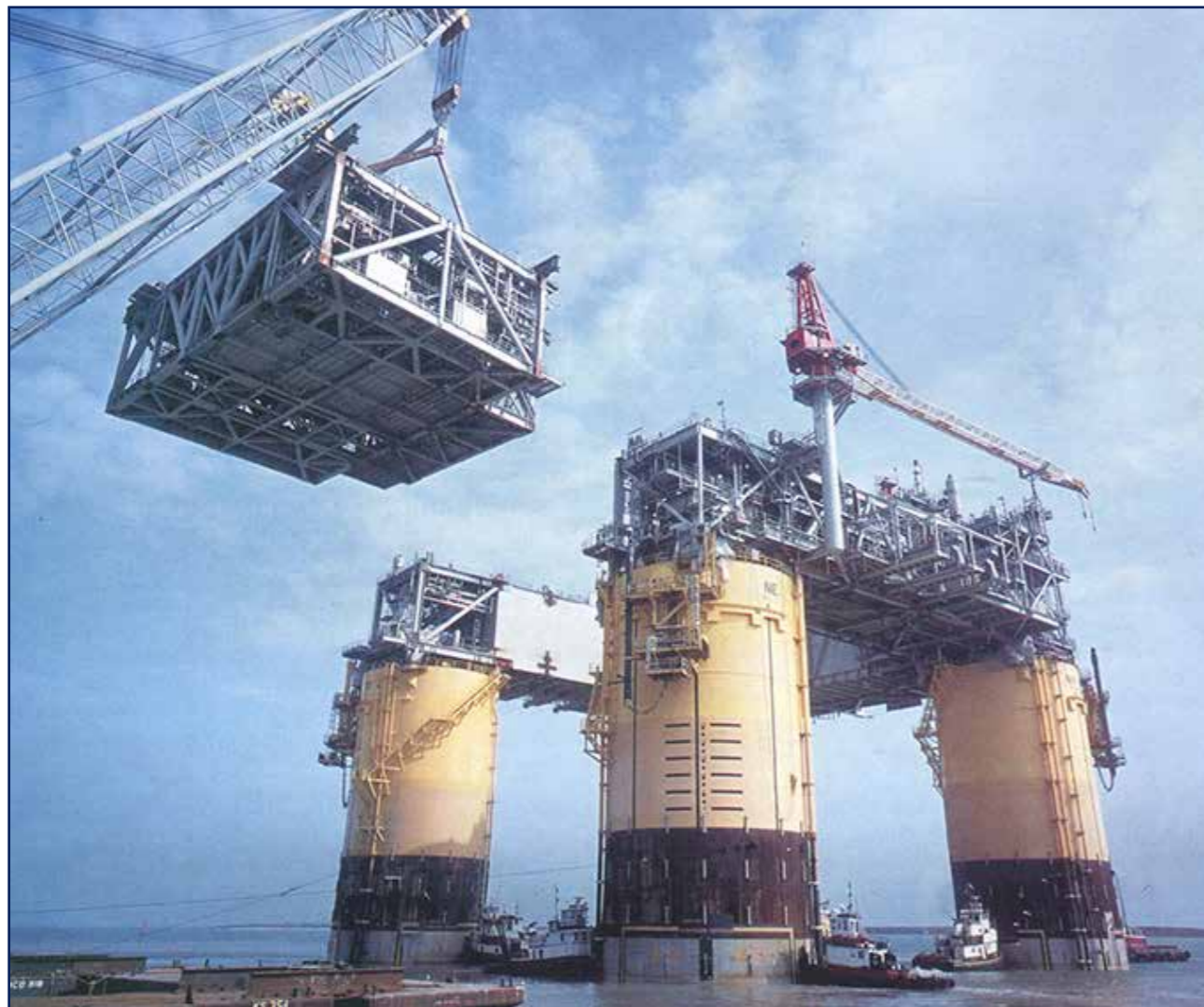
Shell's 5th TLP. It was built at GMF's Ingleside yard to be moored in around 1000m of water. The hull was taken directly from Mars and Ram/Powell while the tendons were taken from Ursa.
