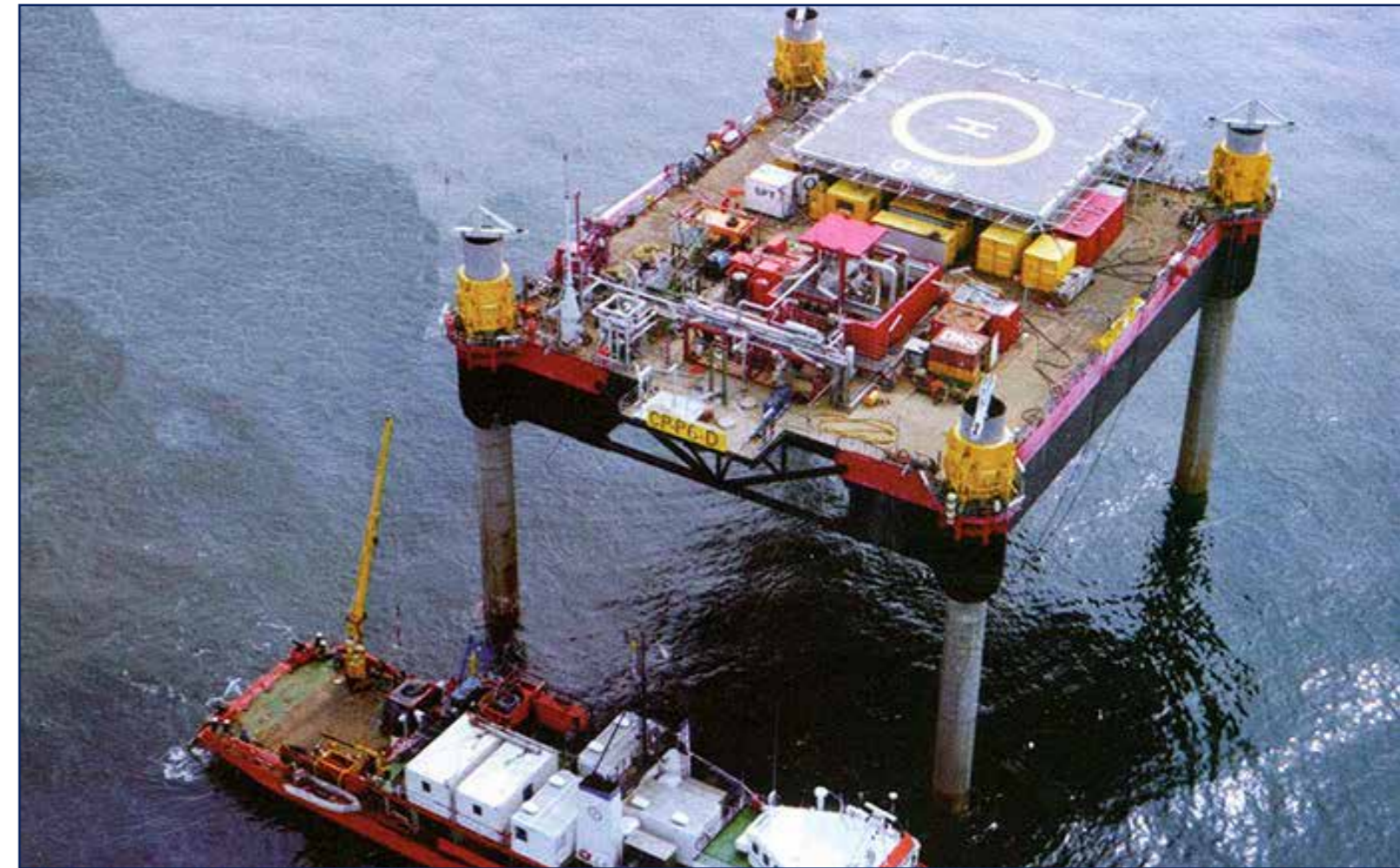
In 2001, KCI Multi Purpose Platforms (MPP) was installed on the Dutch P6-D field. This MPP had previously been producing from the P2-SE field since 1996 and proved that the designs could be re-used.
