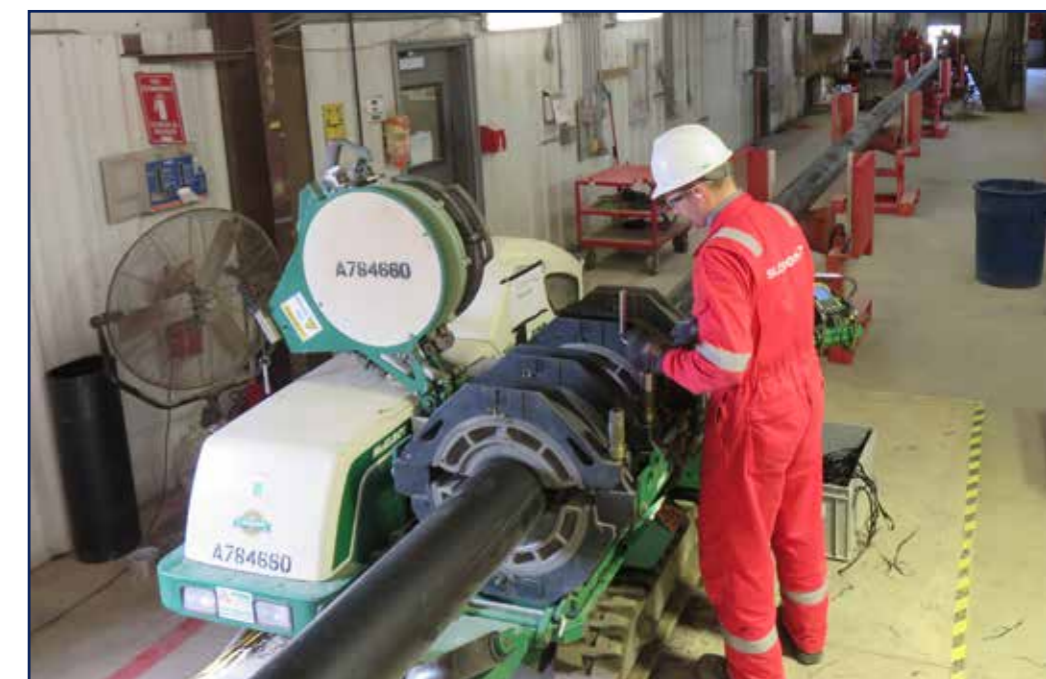
Butt fusion welding of polymer liner pipe
