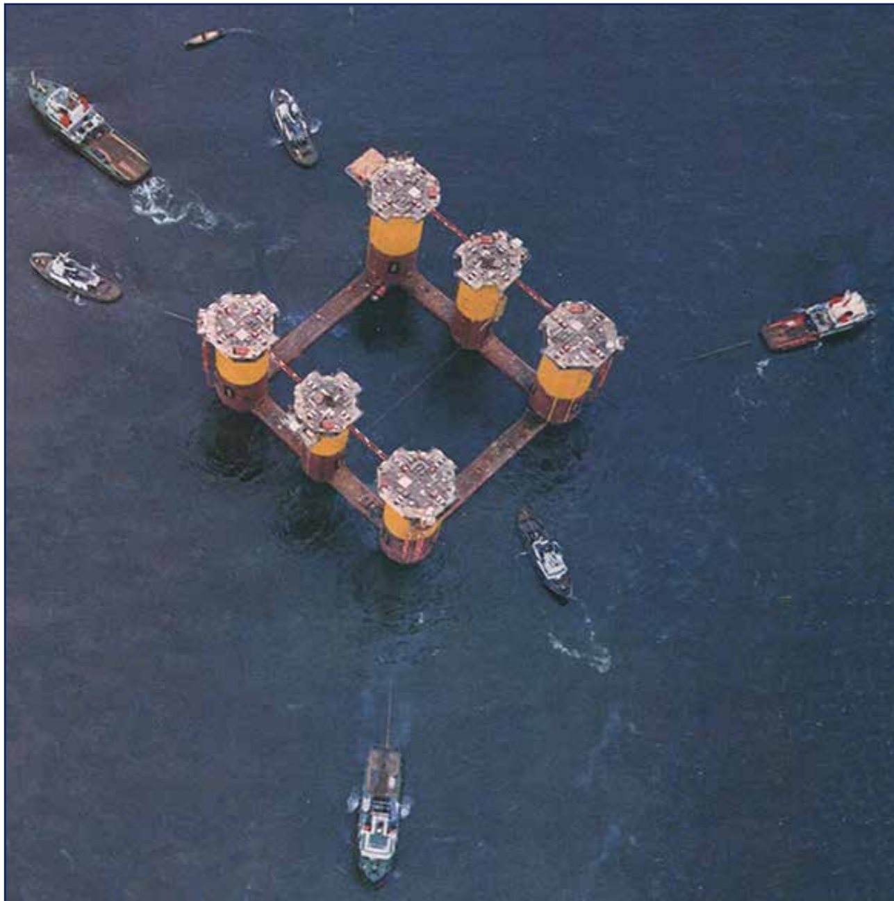
The first TLP hull moves out through the HiFab gates at Nigg and prepares itself for mating with the deck. The topside was built at McDermott's Ardersier yard.
