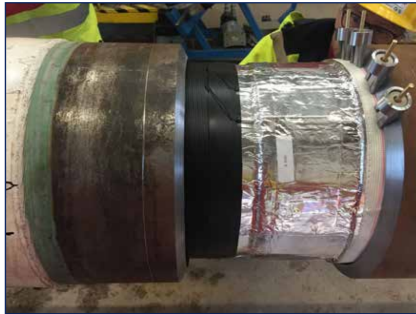
LinerBridge being installed on the firing line
