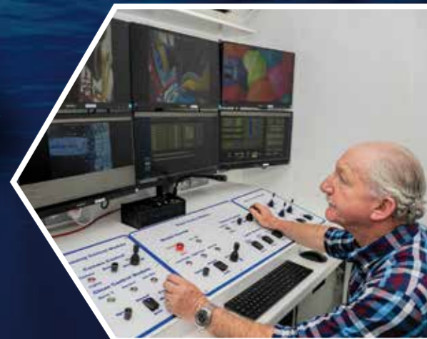
Control Van with screens and controls.
