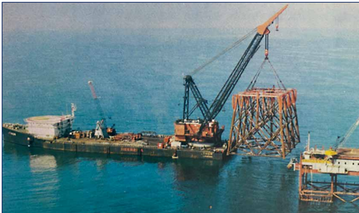
The Thor crane vessel installing the Inde jacket
