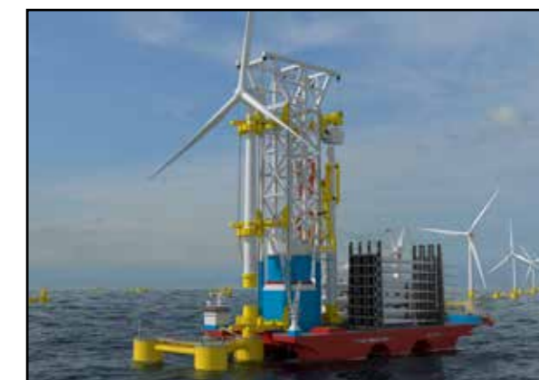
Stabbing the tower onto the floating body
