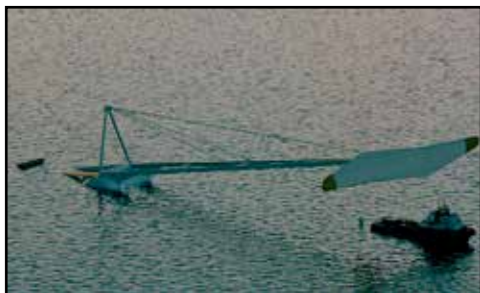
The Touchwind Mono undergoing repairs Touchwind say that a normal turbine costs around €20 million. Their design costs half that.
