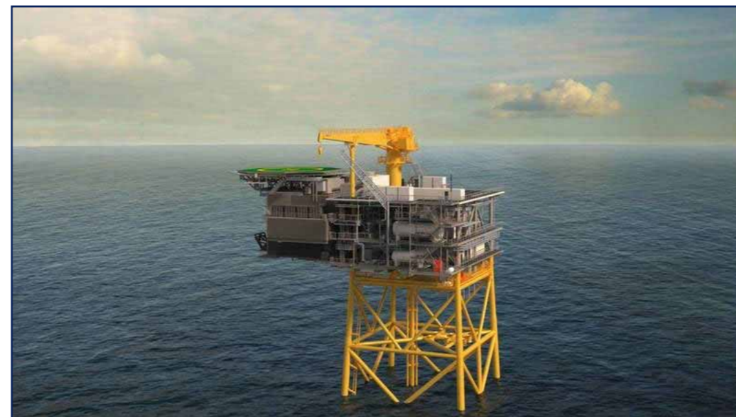
Jackdaw wellhead platform
