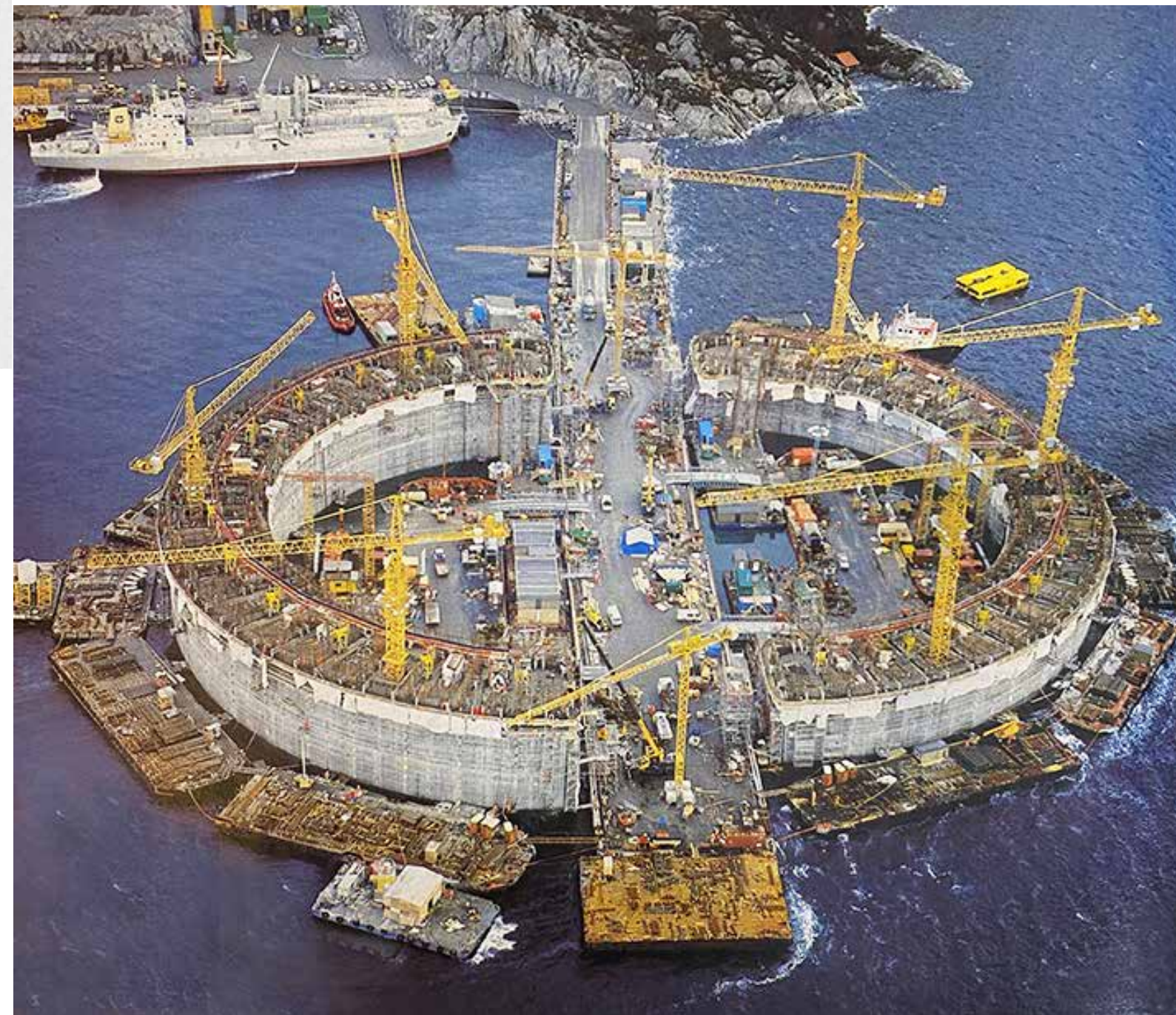
At Alfjord. The two wall units grow at rates of 3m/day.
