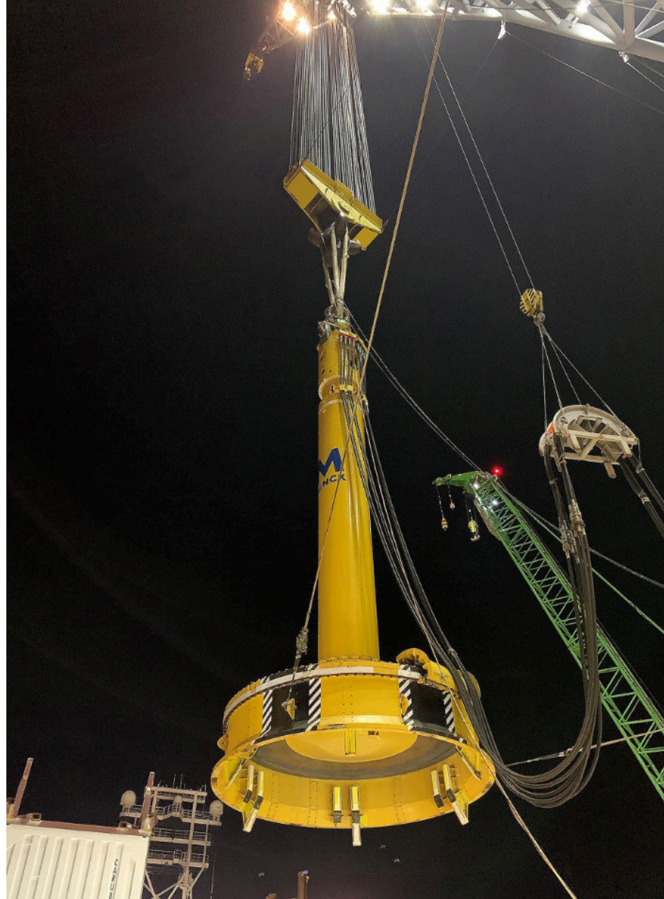
A MENCK hammer being utilised on Vattenfall's Hollandse Kust Zuid I-IV (HKZ) offshore wind farm project in the Netherlands'
