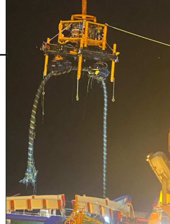
UTROV recovering cable to deck with Multi-Purpose Frame and Grabs
