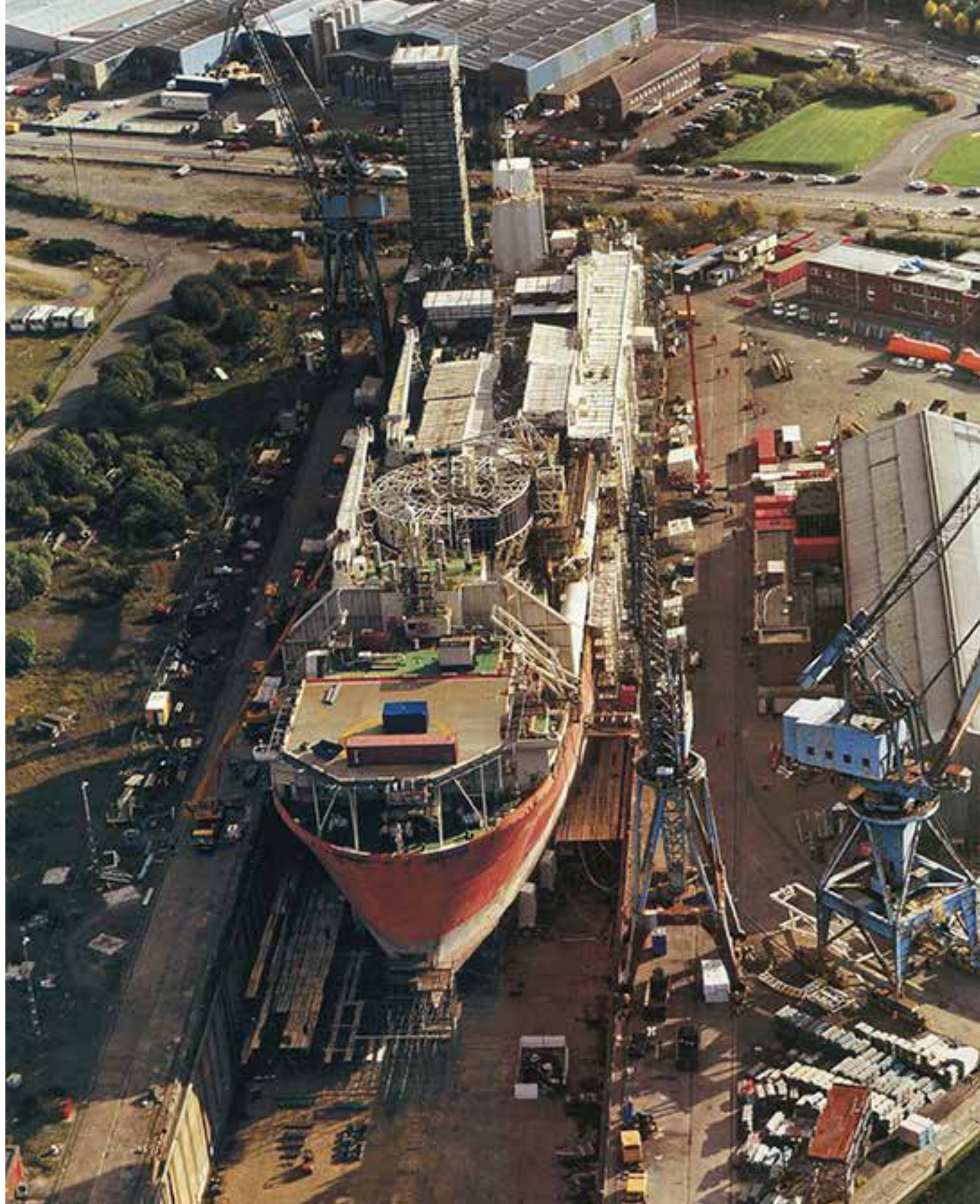
Work on the FPSO at the Inchgreen dry dock by Bouygues Offshore's subsidiary UIE
